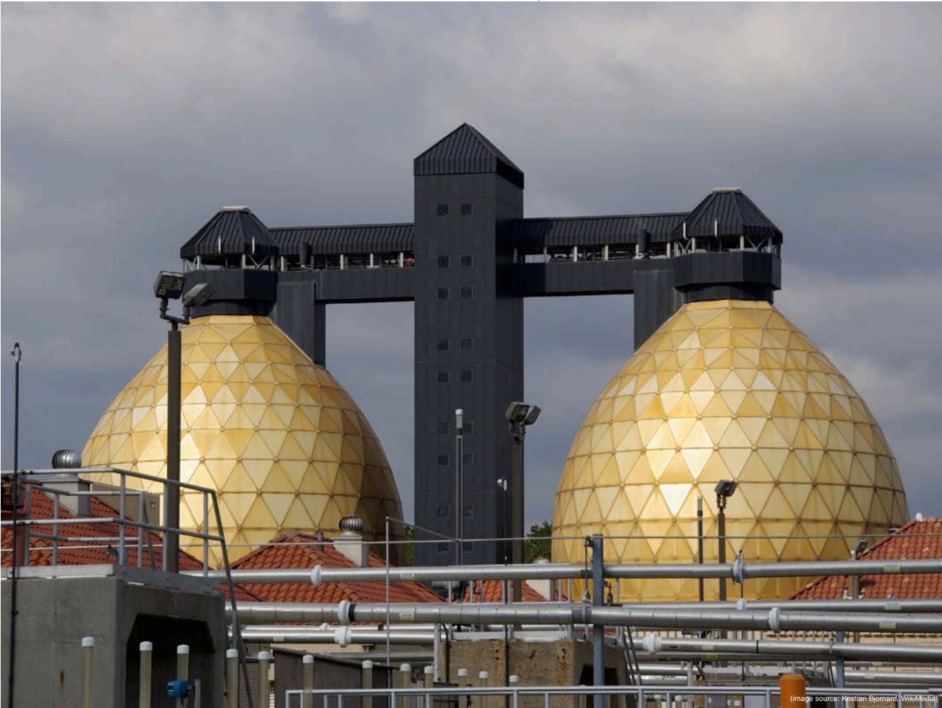
Anaerobic Digesters, Back River WWTW
